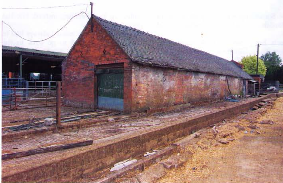
The dairy buildings before and during the transformation
